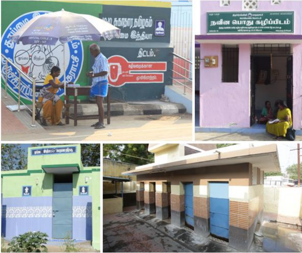
Fig. 9. Public toilets in Tiruchirappalli (Source: TNUSSP)
